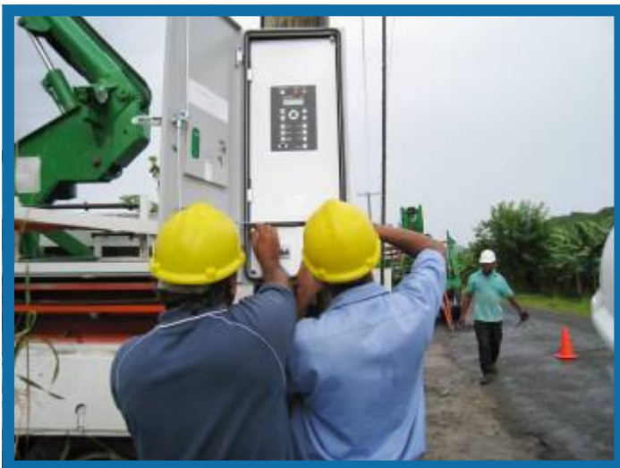
Photos of LUCELEC crew installing an auto-recloser at Vanard. Bottom right: A close-up of the auto-recloser on the pole.
