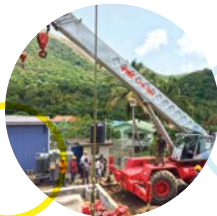
The Soufriere substation was re-commissioned following its shut down in May 2012. Work at the site involved replacing the damaged transformer and upgrading the protection system at the facility
