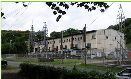
The old Union Power Station will shortly house 2 new high speed units to meet short term capacity requirements
